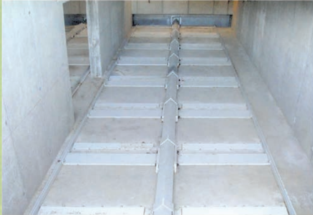
Push rod up to 3 metre width possible per rod
